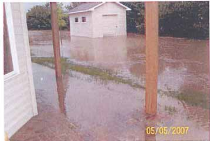
misc flooding 001.bmp
